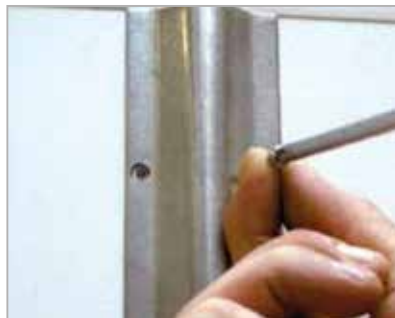
Screw the cable conduit securely in place.
