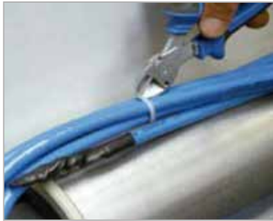
Cut the cable loose with wire cutters.
