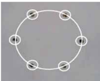
Apply sealant to the liner around and between the holes.
