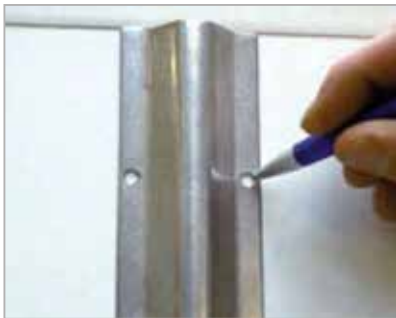
Mark the mounting holes and drill them.
