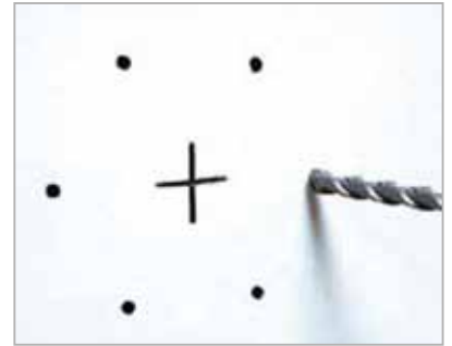
Drill holes with \varnothing 11 mm bit. At least 80 mm deep.
