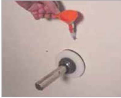
Fully insert funnel pouring hose into pouring channel.
