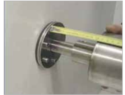
Determine length of spacer bush and cut to length.
