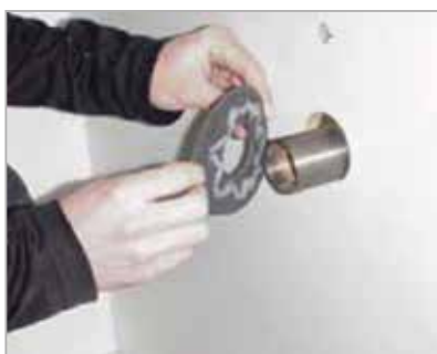
Fit gasket with sealant in motor well.
