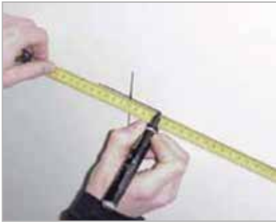
Mark the dimensions of the wall duct.
