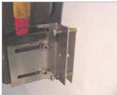
Slide plugs into drill holes and drive in with a bench hammer until bolt head touches bracket.
