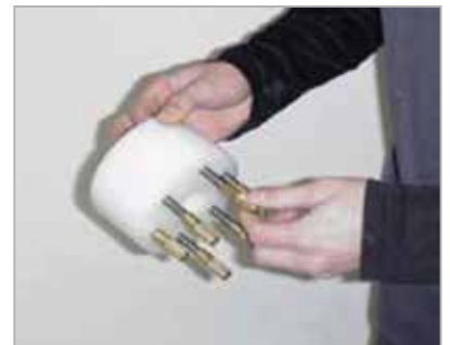
Place plugs on tap bolts and tighten to expansion slug.
