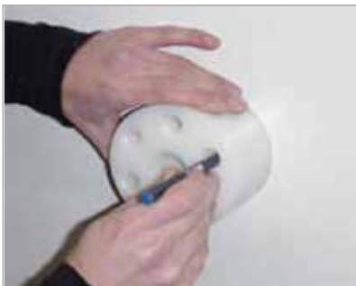
Insert plug, place bearing block and mark remaining holes.
