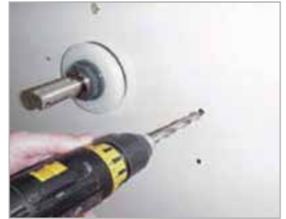
Drill \varnothing 11 mm holes, at least 80 mm deep.
