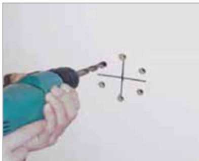
Remove bearing block and drill remaining holes.
