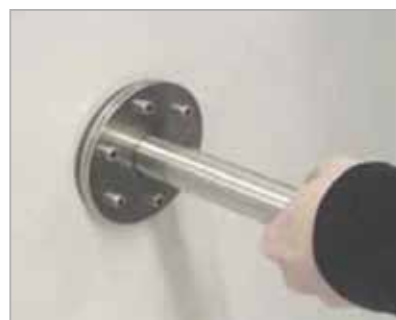
Fit the drive shaft.
